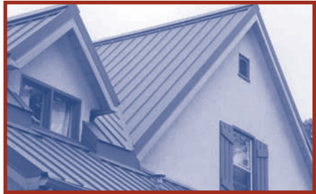
Metal, tile, asphalt, ULC-rated treated shakes or non-combustible material (0 pts) - the most fire resistant and remain effective under severe fire exposure.
