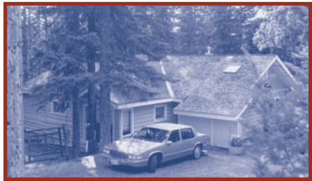
Unrated wood shakes (30 pts) - provide no fire protection.
