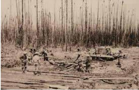
Figure 12: A corduroy road under construction through a very swampy black spruce lowland
