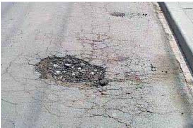
Figure 19: Potholes such as this can damage vehicles, and each year millions of dollars are spent repairing them.
