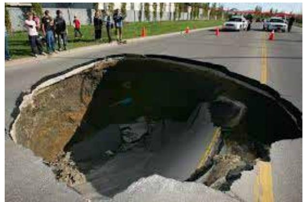
Figure 19A: Sometimes a pothole can continue to grow until it forms a sinkhole. Sinkholes can create serious public safety issues.
