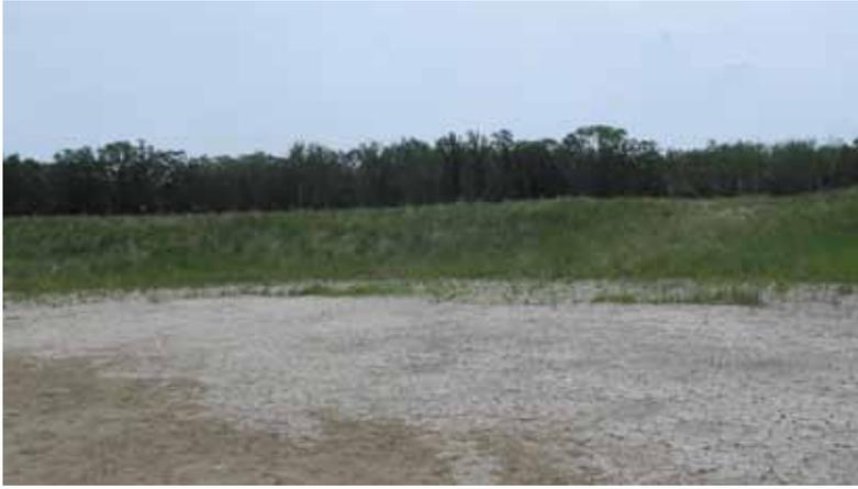
Figure 23: The Lafarge quarry in the Stonewall area is being actively mined, and rehabilitated at the same time. The walls of the quarry are gently sloped and seeded with grasses and alfalfa to prevent erosion. The image shows only 1 year of re-growth.
